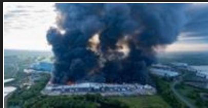
E-comm. Warehouse Fire (UK, 2021)
