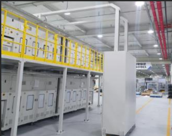
Pre-charge S/C installation
