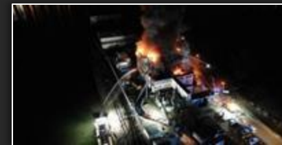
Data Center Fire (France, 2021)
