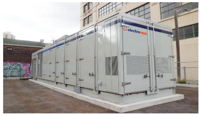
Energy Storage System installed at Ryerson University in Downtown Toronto
